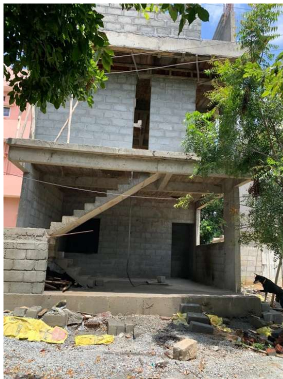
A House under Construction in Mathrudhan
